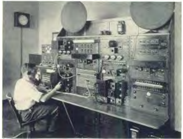
Control room adjacent to studios, where operator measures and amplifies programs telephoned to plant.
