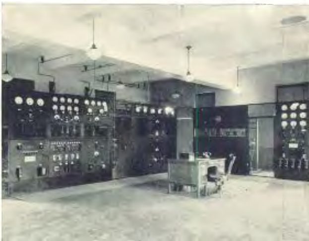
Transmission room with compact panel arrangement which permits one operator to observe all operations.
